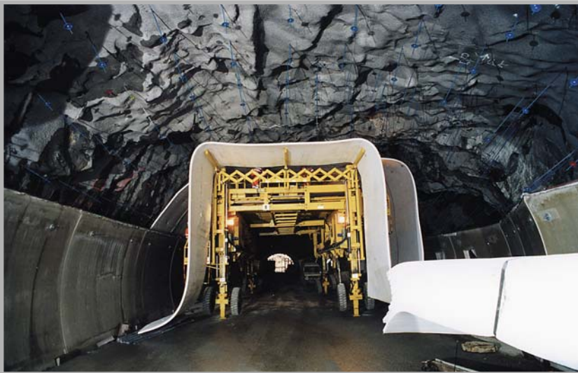
Pre-fabricated concrete and PE foam
