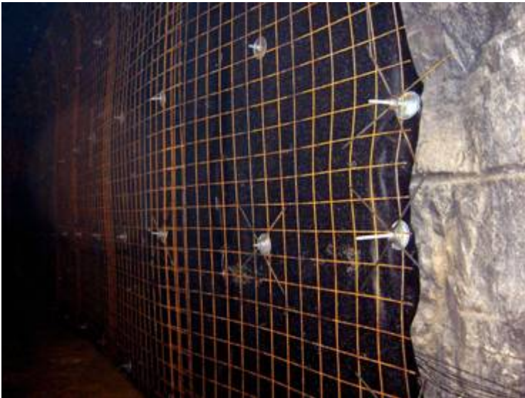
Mesh reinforcement combined with membran and sprayed concrete
